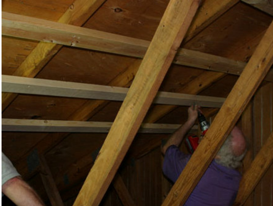
Figure 17. Installation of upper horizontal brace.
